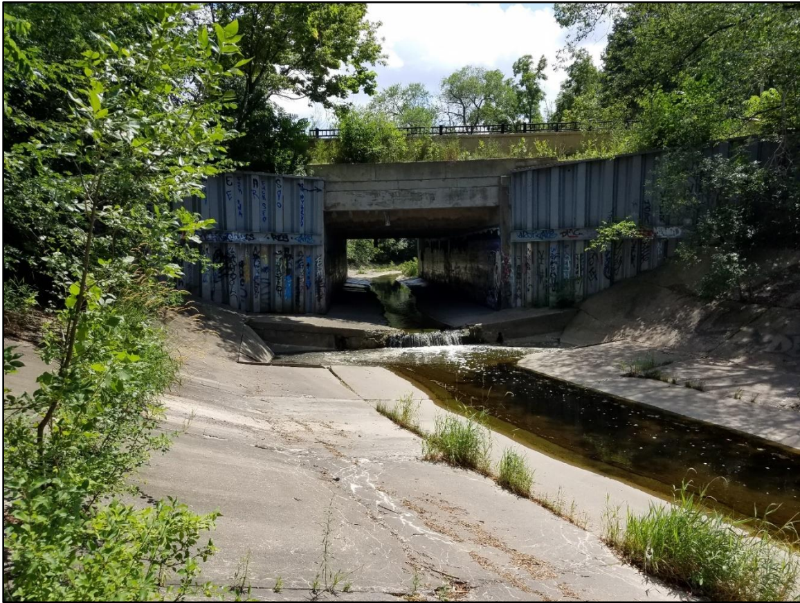
Figure 13: Channel Conditions Downstream of Bridge
